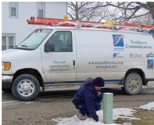
Adam removes the snow from around one of Northwest's telephone pedestals prior to performing maintenance.
